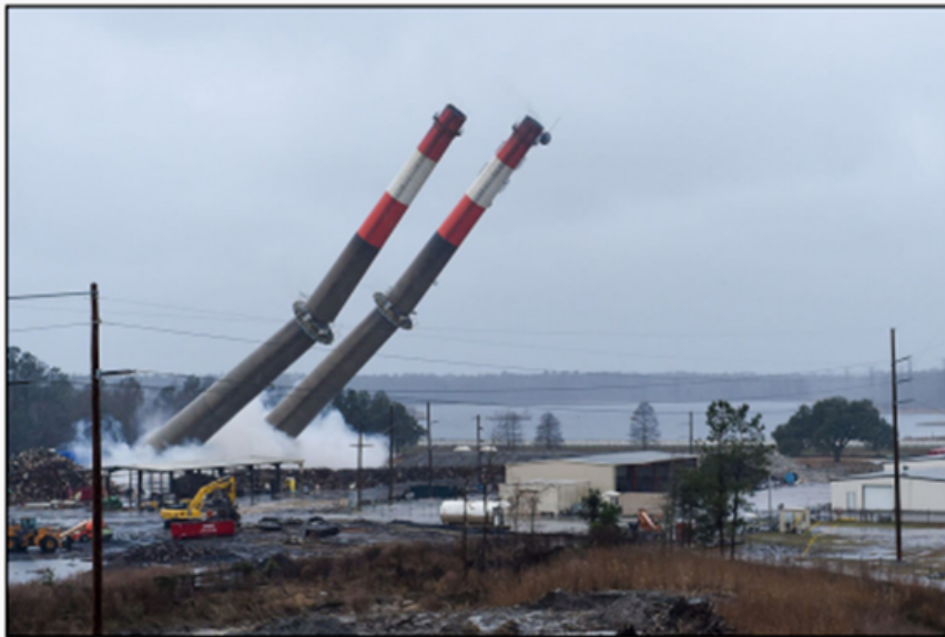
Demolition of the Grainger Generating Station stacks
